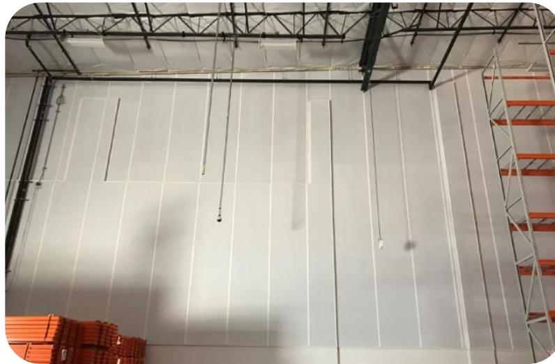
Quick Clip seals seams between insulation panels.
