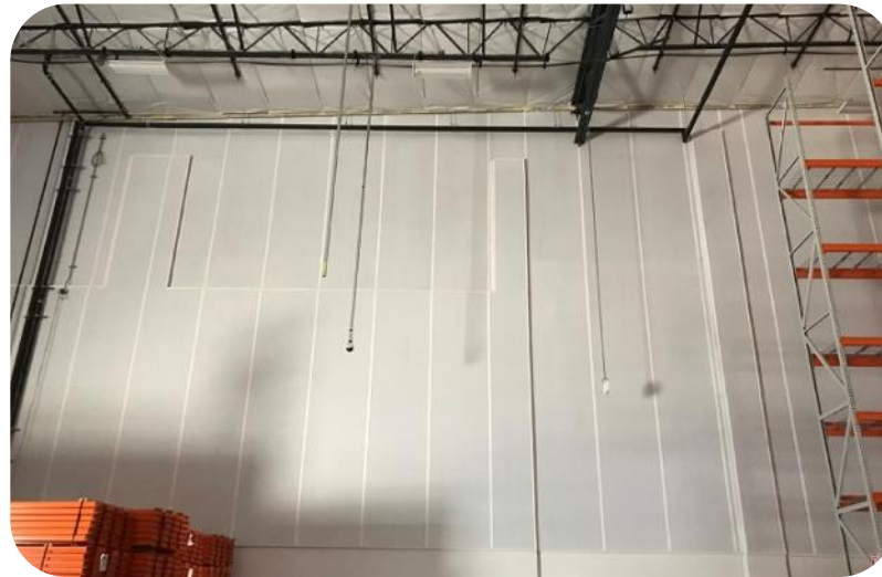
Quick Clip seals seams between insulation panels.
