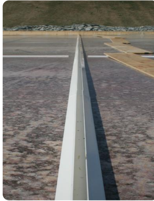
#767 Standard Series Bulkhead attached with #876 Base Clip
