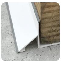
Rigid PVC structure provides a superior finish, while the flexible PVC seal eliminates the need for caulking.
