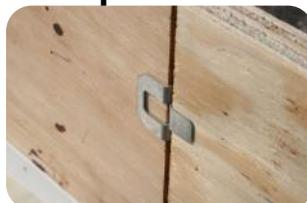
**Step 6** - Use an H style roofing clip between each section of lumber to align.
