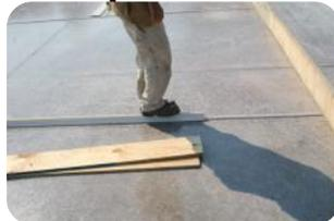
**Step 3** - Continue pressing the entire length of the Bulkhead into the Base Clip.
