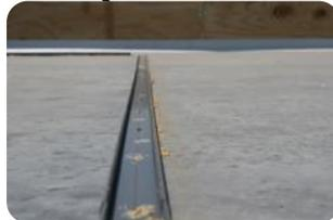
**Step 2** - Press one end of the Bulkhead's interlocking teeth into the end of the Base Clip.
