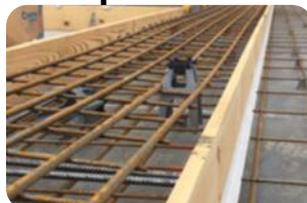
**Step 5** - Using a 1" board, apply downward pressure in the channel of the Bulkhead, working from one end to the other until it is seated in the channel. This creates a tight friction fit with the board, preventing it from rising during the pour. No nailing is necessary.
