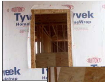
Raw Window Opening
