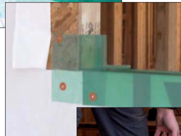
Secure with Nails or Staples
