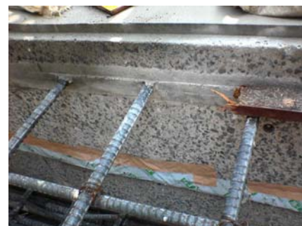
Retamate was used to prepare a concrete joint.
