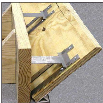
Assembled Miter Corner Brackets and Chamfer
